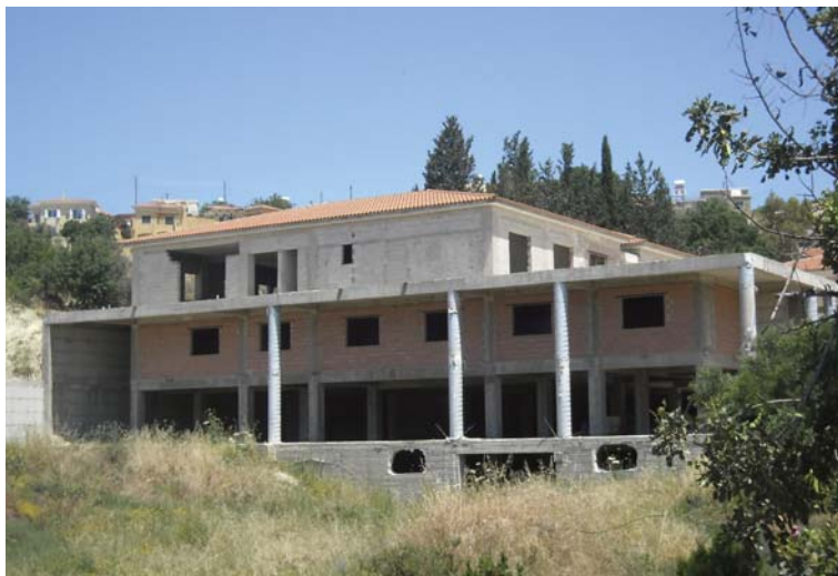
● Saint Michael's Hospice under construction in Mesa Khorio.
